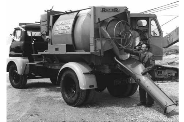
Lorri goncrit Ready-mix
